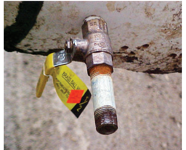
Obtaining a representative sample of liquid manure or slurry can be challenging. Most labs prefer that liquid samples fill the bottle to within an inch of the top. Installation of sampling ports with an attached hose can make sampling events much more pleasant.
