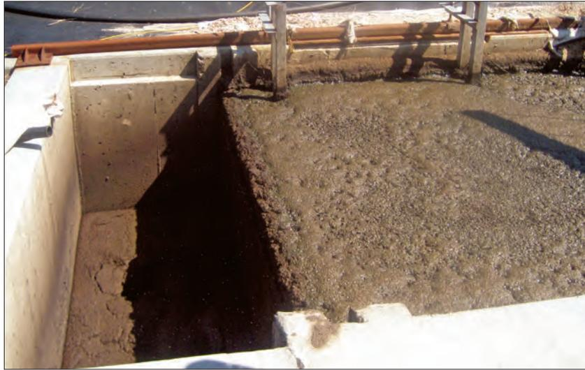
In a two-stage anaerobic manure digestion system the process is separated into distinct portions, mirroring the biological process. High solids waste are placed in a concrete bay where water is passed through, effectively leaching out organics that are later converted into methane gas.
